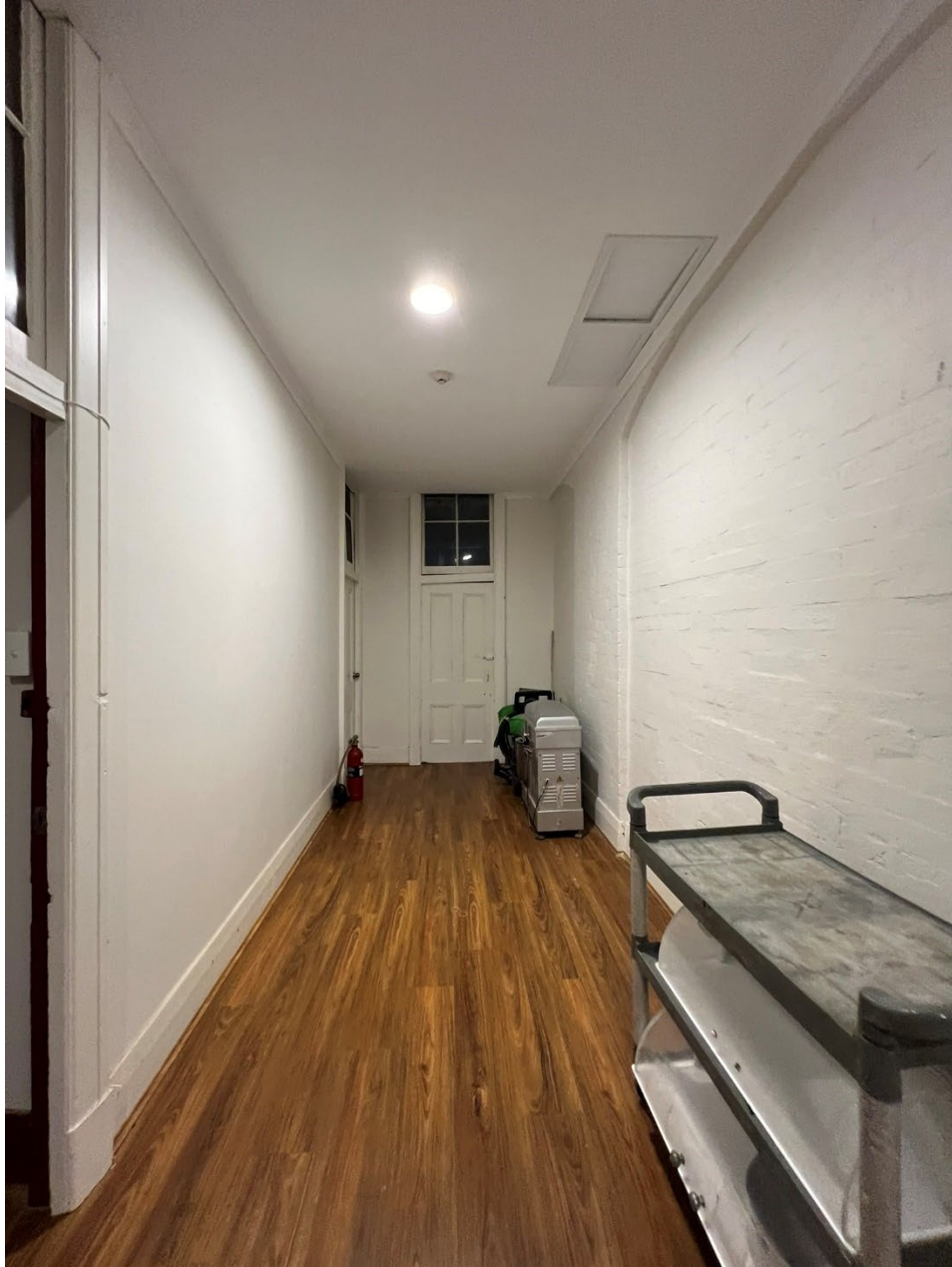
Figure 46 Second floor with 100 Hay Street with original joinery and recessed brick arches, false ceiling and modern floor boards.
