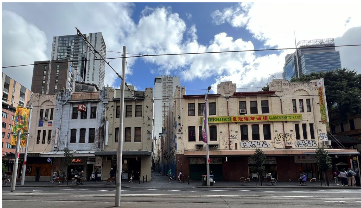
Figure 35 Nos. 90-100 Hay Street with Kimber Lane traversing between nos. 94 and 96.
