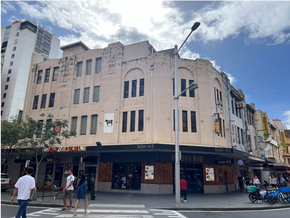
Figure 36 No. 90 Hay Street with its chamfered corner, arches and pointed parapet.
